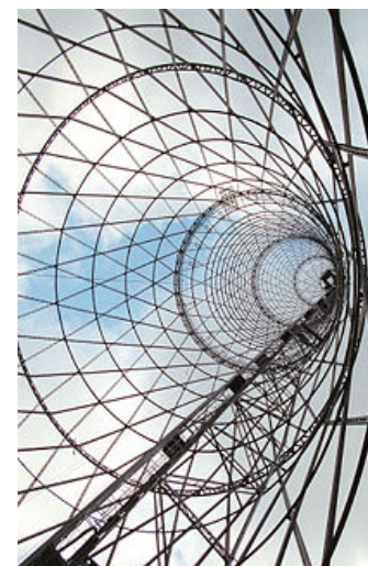
The Hyperboloid lattice shell of Shukhov Tower in Moscow, Russia.
